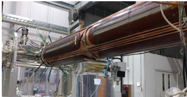
Installation of water jacket (bottom side)
