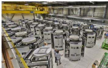
CERN 160 kW @ 200 MHz 2021 Power density 15 \text{ kW m}^{-3}
