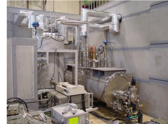
J-ADS 972MHz Cryomodule
