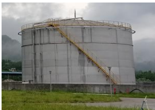
5000 m 3 LAB storage tank
